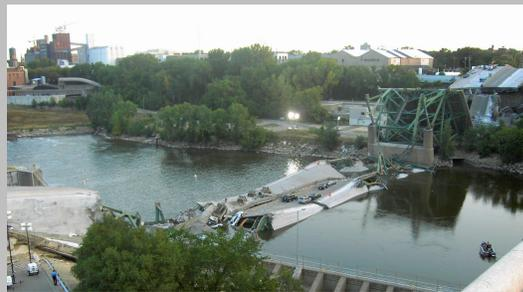
*Figure 1.1: During the evening rush hour on August 1, 2007 the I-35W Mississippi River bridge collapsed killing 13 people. Federal inspection had ranked the bridge structurally deficient, like about 70,000 other bridges in the U.S.*
